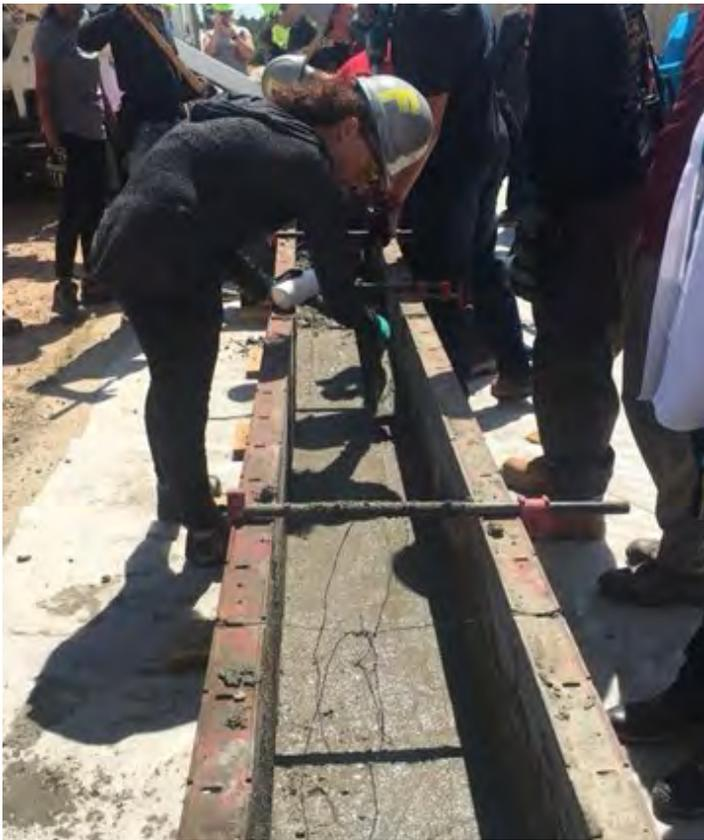
Photo Above: Madigan Kinsey performing finish work on a concrete beam .
